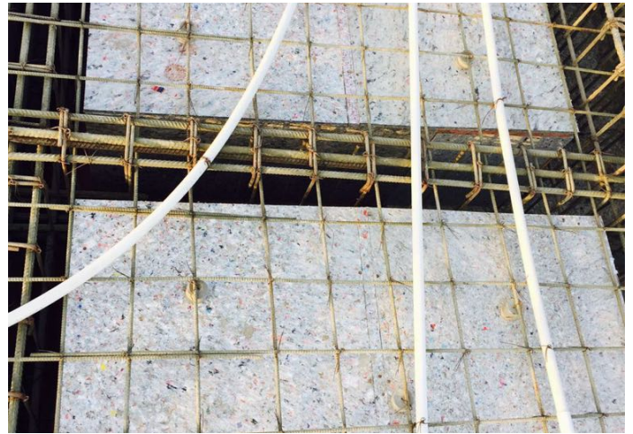
PANELS IN SLAB FORMWORK
