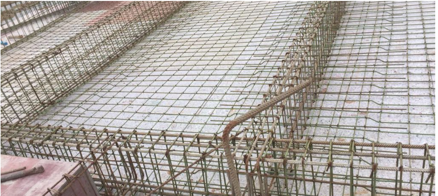
PROJECT PHOTO / Slab decking and beam reinforcement
